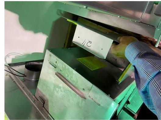
Figure 2: 2" Return Inlet Retrofit Piece
