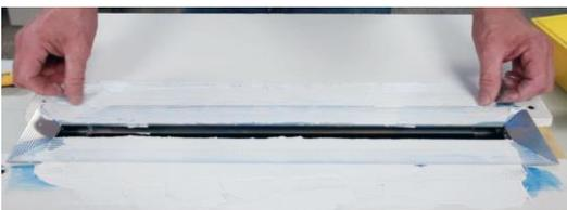
Apply second coat of drywall compound over tape and smooth. Allow to dry.
