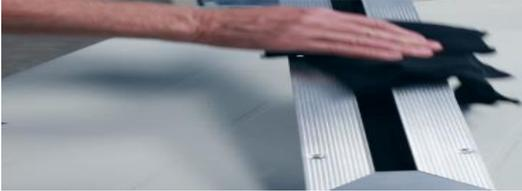
STEP 2: Apply one coat of **bonding agent** that is compatible with plaster over entire surface of flange, and allow to dry as per manufacturer's instructions.
