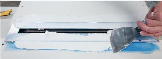
STEP 4: Apply a 4" **wide mesh or paper tape to joint compound**. Be sure to smooth out and remove air pockets. Mesh or tape should cover diffuser flange, but not the inside vertical edge of diffuser frame.
