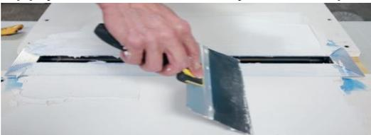
STEP 5: Apply at least two coats of finishing compound. Allow to dry. Afterwards, sand smooth, prime, and paint surface.
