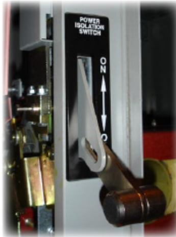
Figure 4: 4160V Isolation Switch
