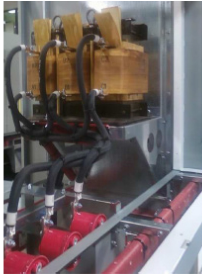
Figure 6: Typical Output Reactor
