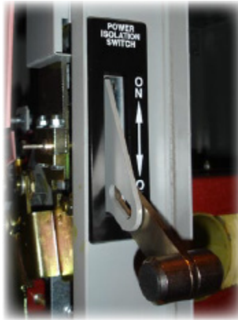
Figure 4: 4160V Isolation Switch
