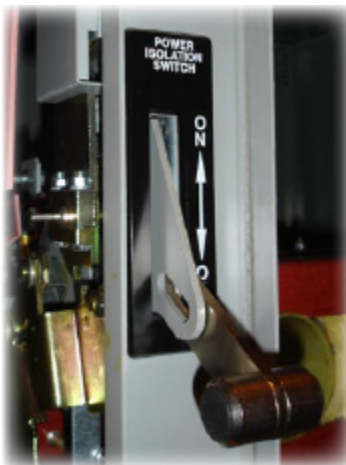
Figure 4: 4160V Isolation Switch
