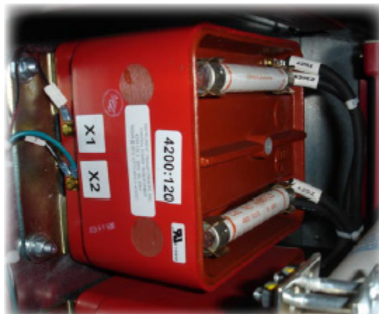
Figure 3: Typical Control Power Transformer
