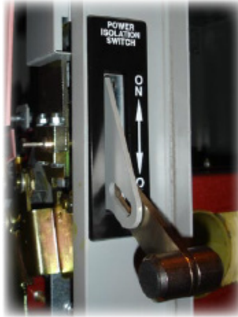
Figure 4: 4160V Isolation Switch
